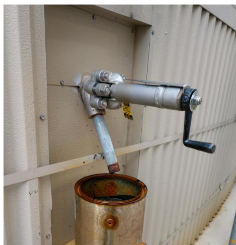
Figure 1 Examples of Valves Commonly Used for Sampling Liquid Asphalt from Tanks
