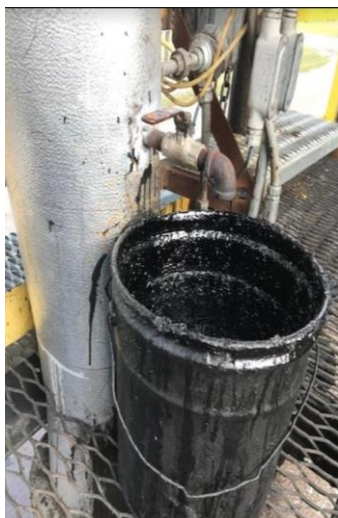
Figure 4 Examples of Valves Commonly Used for Sampling Liquid Asphalt from Pipelines
