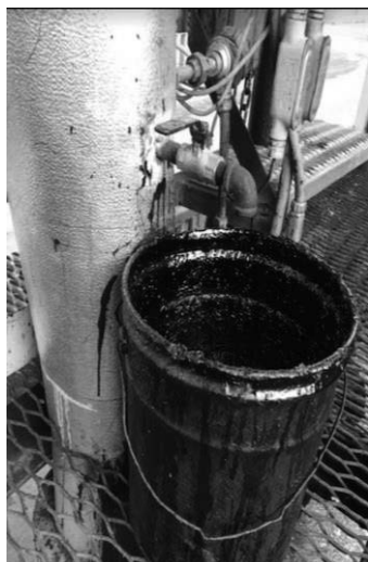
Figure 4 Examples of Valves Commonly Used for Sampling Liquid Asphalt from Pipelines
