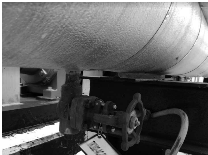
Figure 4 Examples of Valves Commonly Used for Sampling Liquid Asphalt from Pipelines
