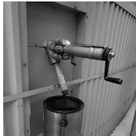
Figure 1 Examples of Valves Commonly Used for Sampling Liquid Asphalt from Tanks
